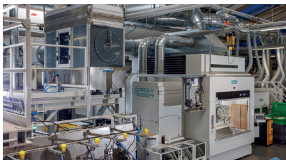
Recirculating air/humidification Unit
